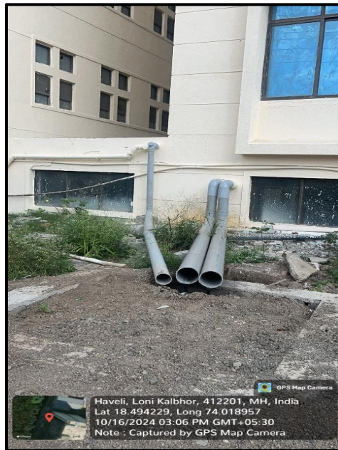
Building: IT Building
