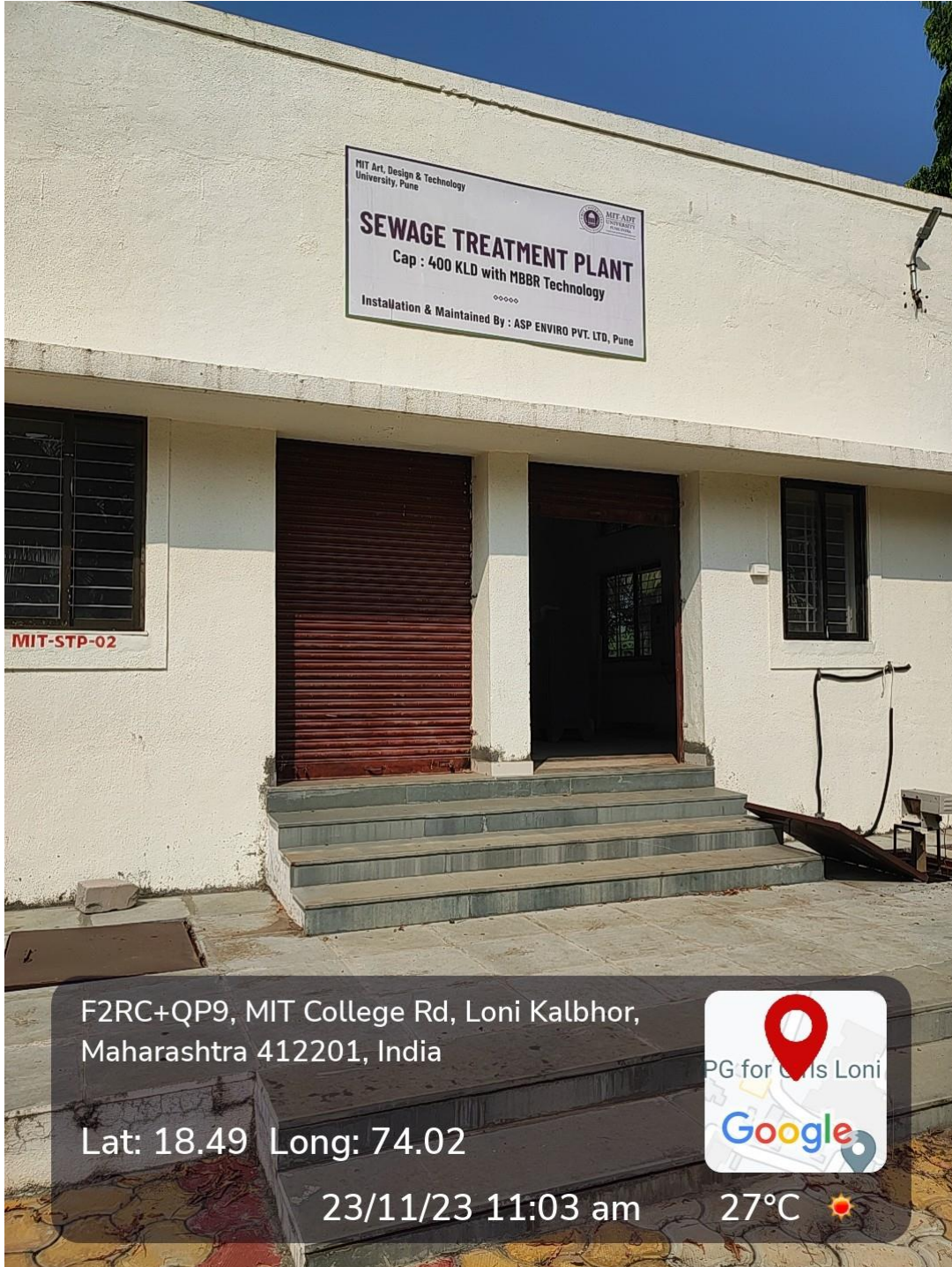
Geotagged Photograph of Sewage Treatment Plant
