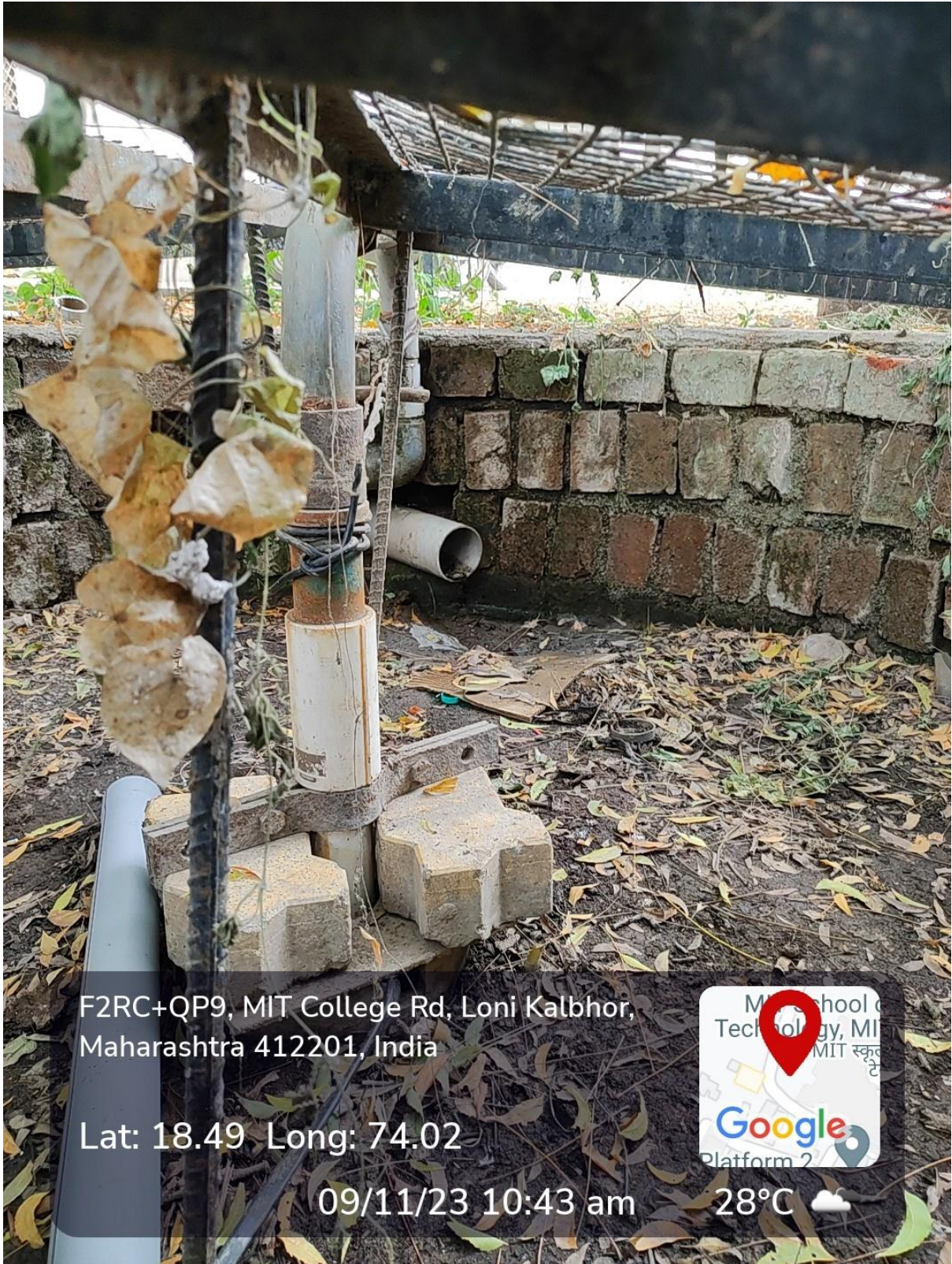
Geotagged photograph of Borewell Recharge
