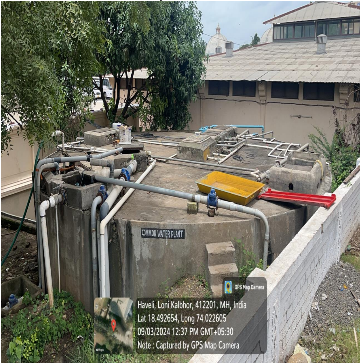
Geotagged Photograph of Water Tank
