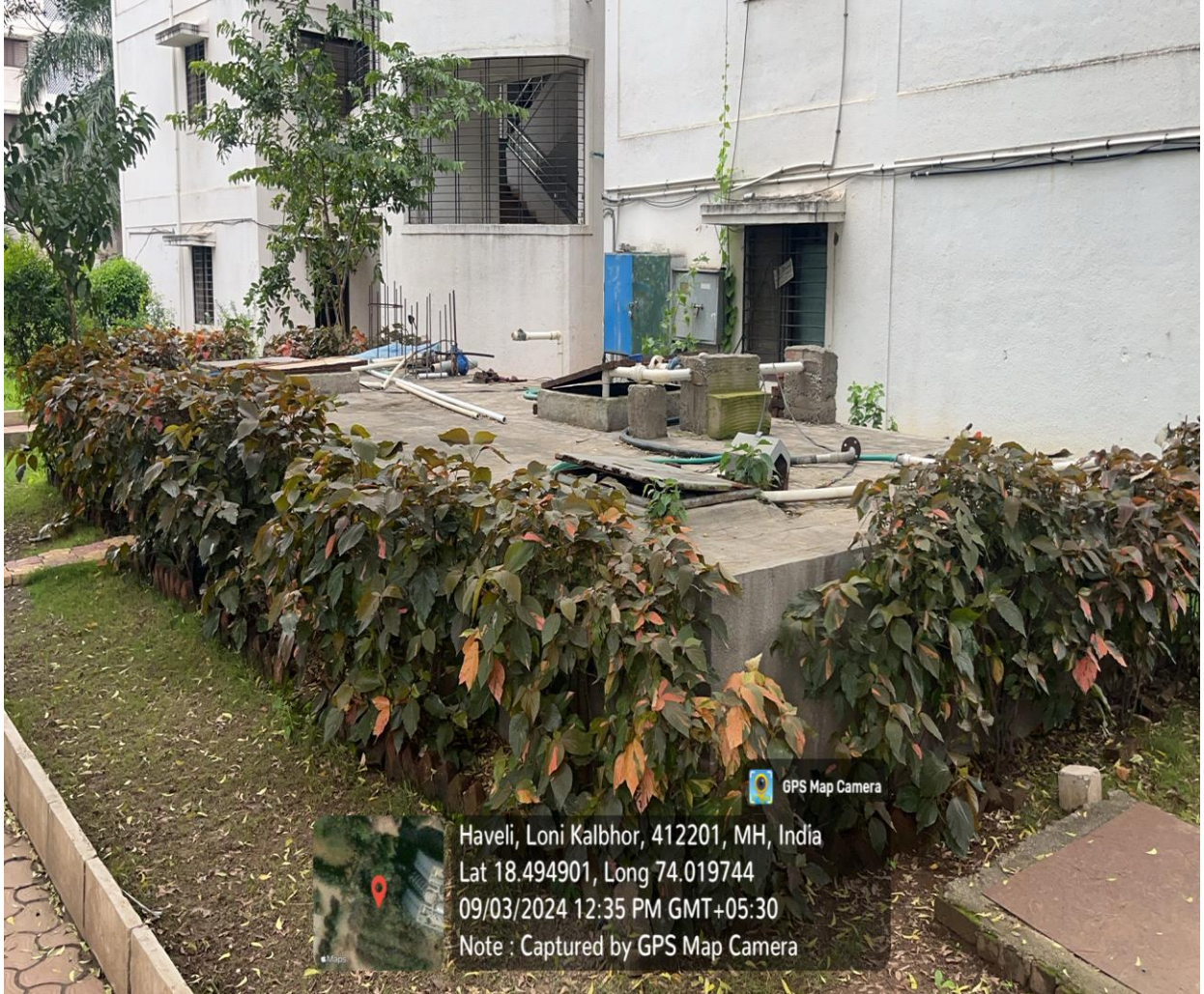
Geotagged Photograph of Water Tank
