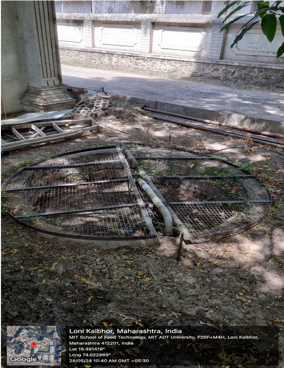
Geotagged Photograph of Borewell Recharge
